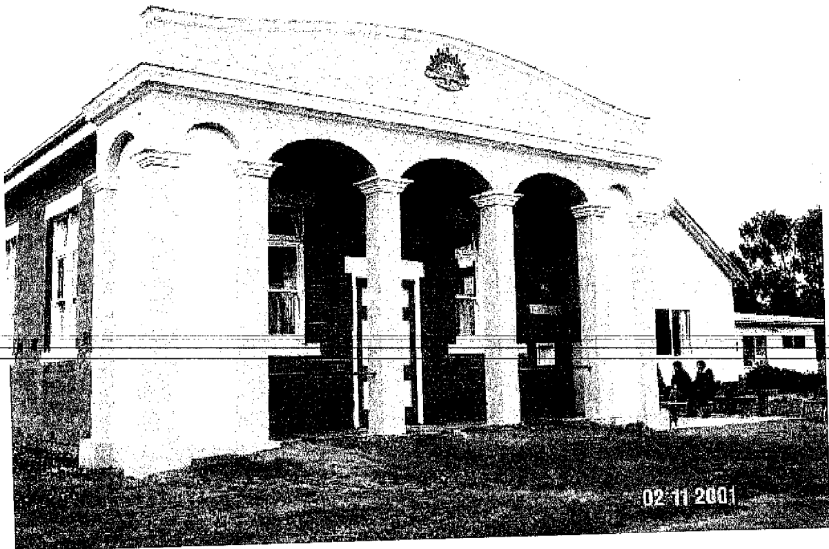
Cavendish Memorial Hall, Barker Street, Cavendish
