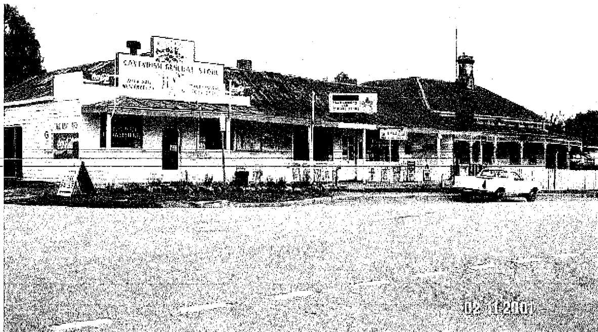
Cavendish General Store & Residence
