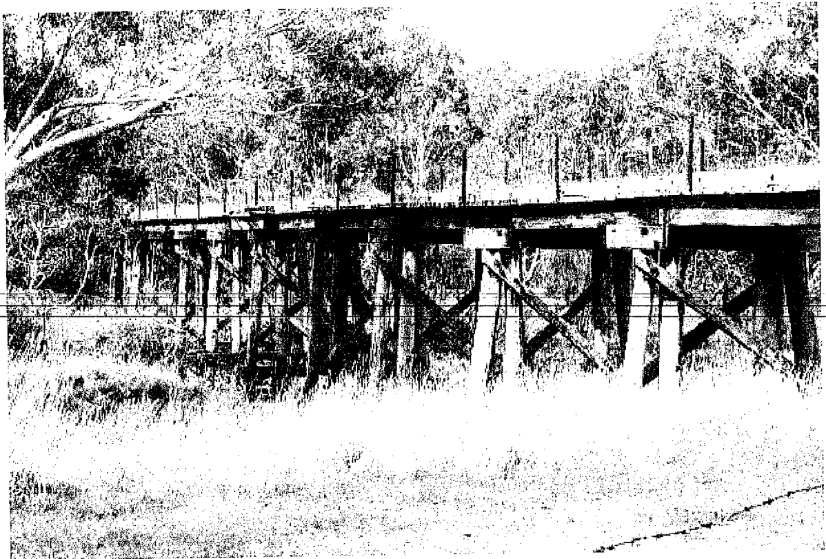
Railway Trestle Bridge, over the Wannon from the east
