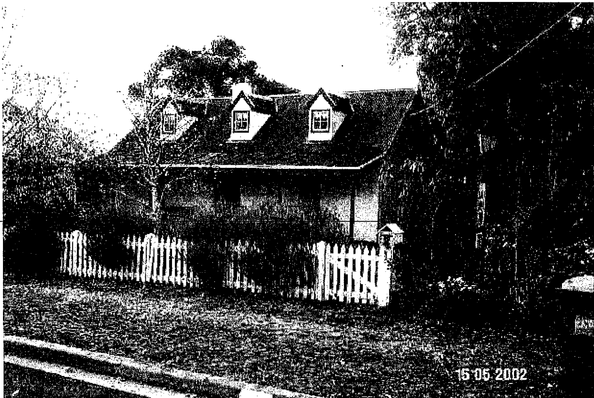
Lutheran Manse (Former), 8 Hiller Lane, South Hamilton
