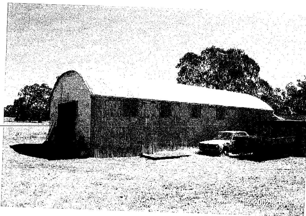
Pre-fabricated Shed, Indi Homestead, Balmoral
