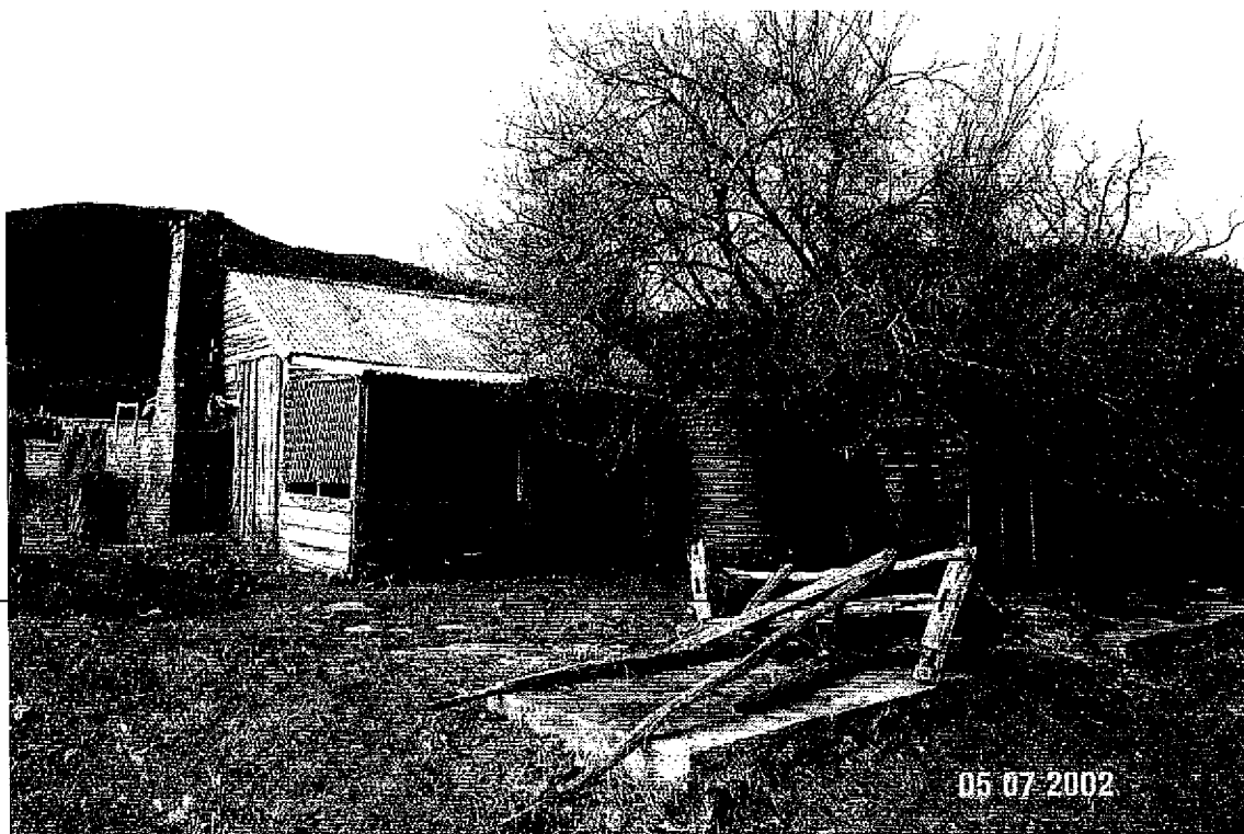
Rosebank Homestead, Neate's Road, Victoria Valley
