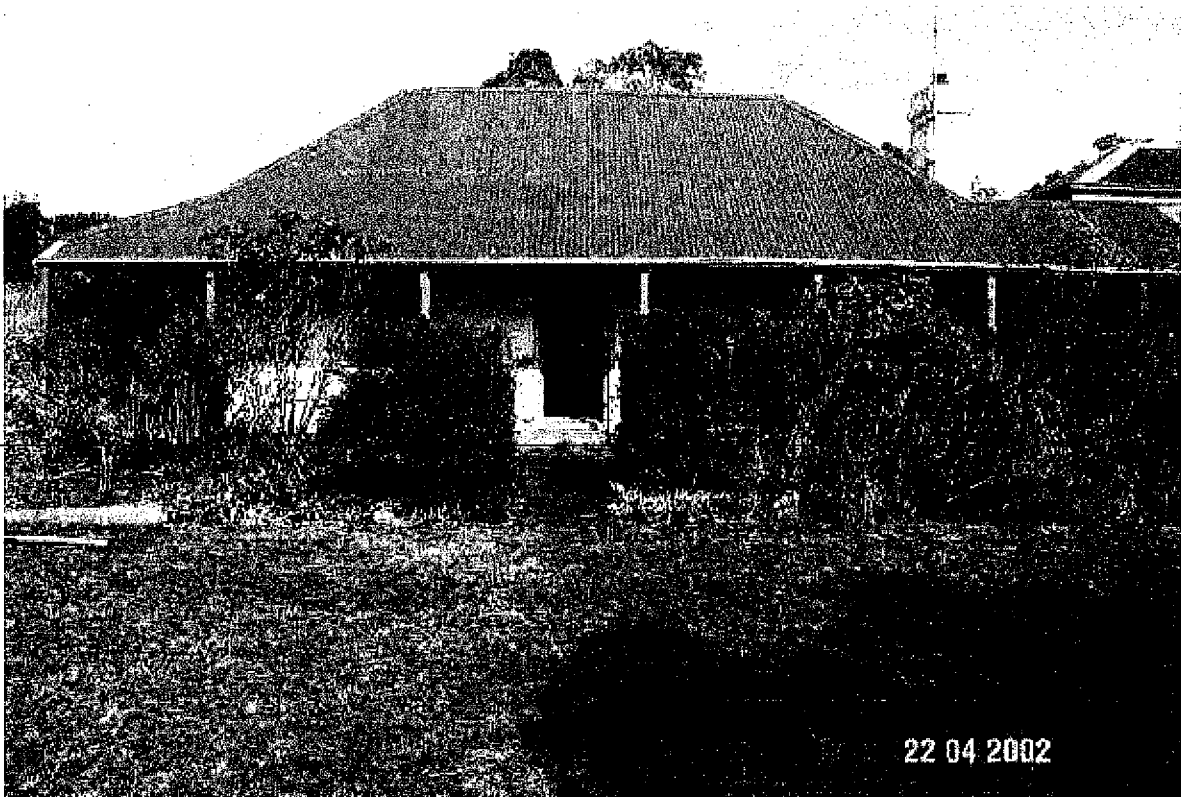
Aitkin's Wattle and Daub Cottage, 57 Bell St, Penshurst
