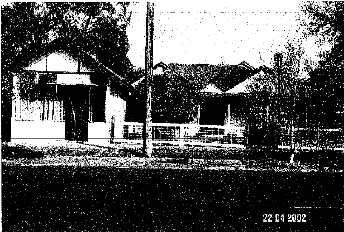
Common School (Former) and Shop, 83a-b Bell St, Penshurst
