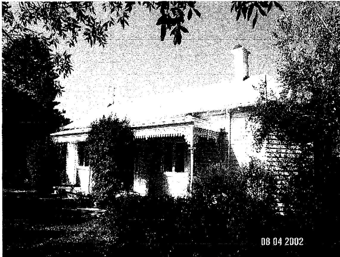
Aird, Sutties Road, Byaduk. Façade.
