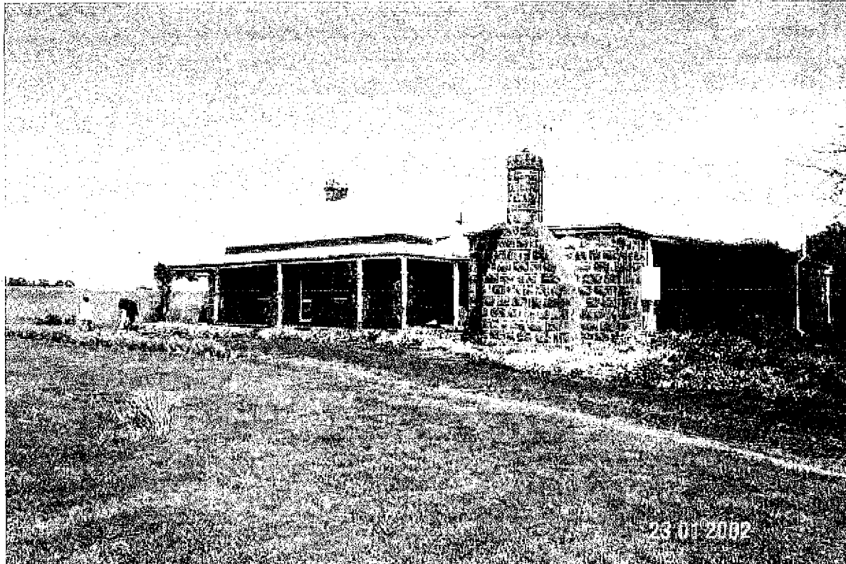
Lyne Homestead, Branxholme-Byaduk Road, Byaduk North, side elevation
