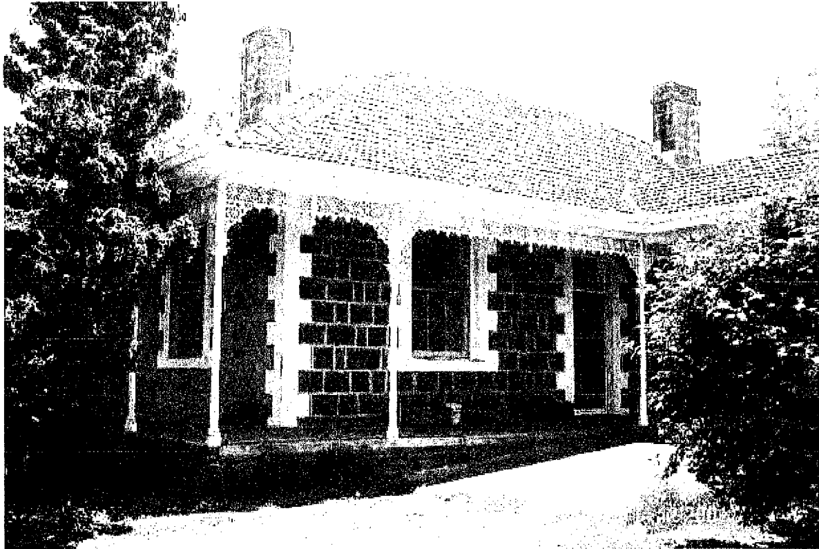
Brisbane Hill Homestead, North Verandah, Hamilton - Port Fairy Road, Byaduk North.
