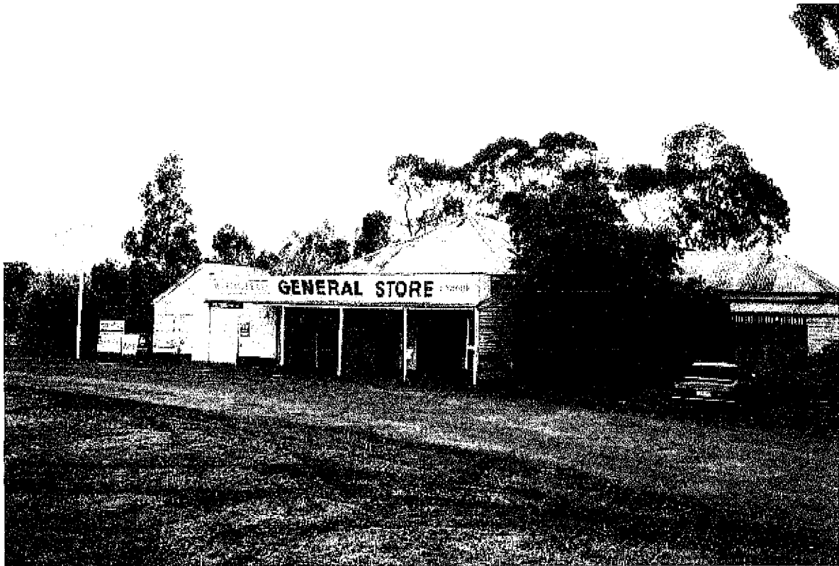
General Store and Residence, Port Fairy - Hamilton Road, Byaduk
