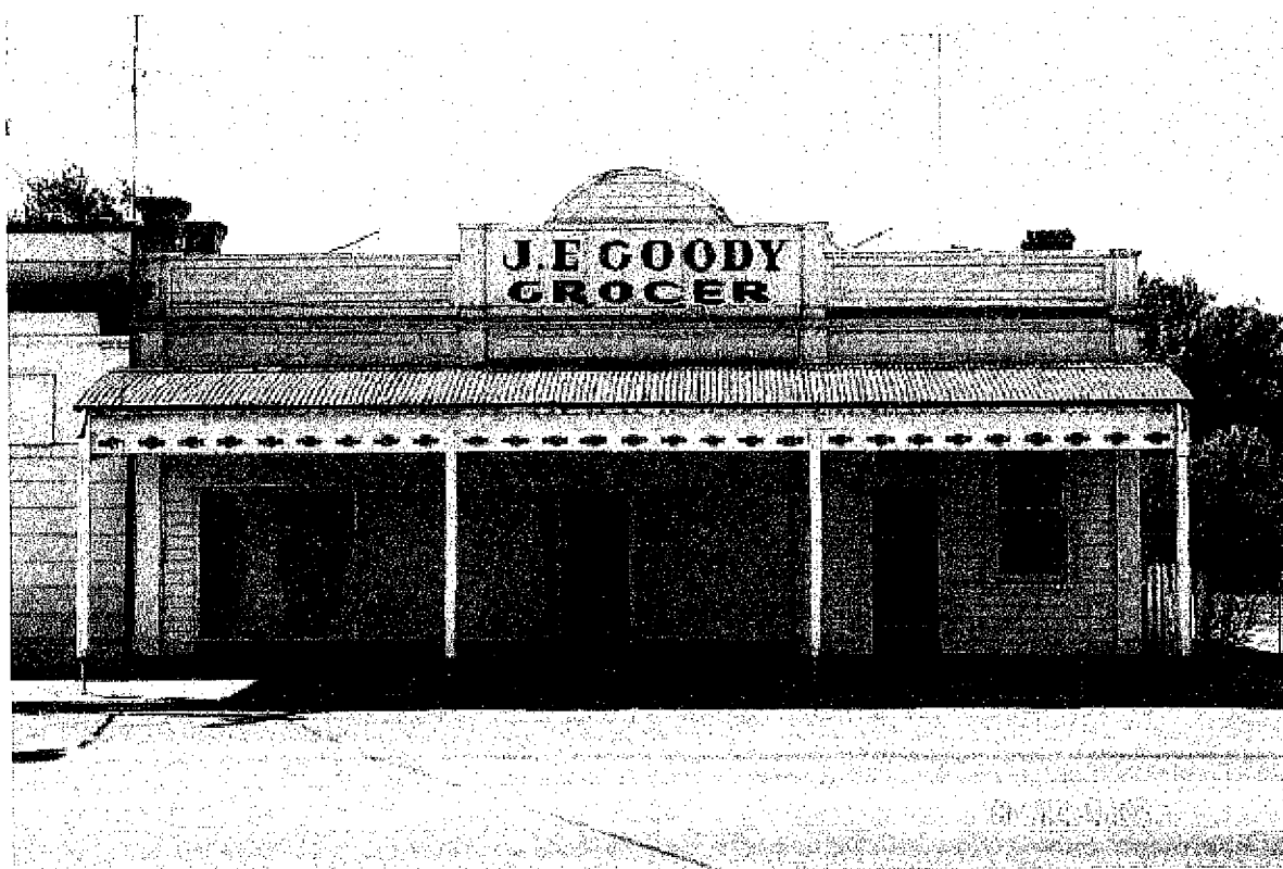
J. E Goody's Store and Residence (former), Whyte Street, Coleraine. Façade
