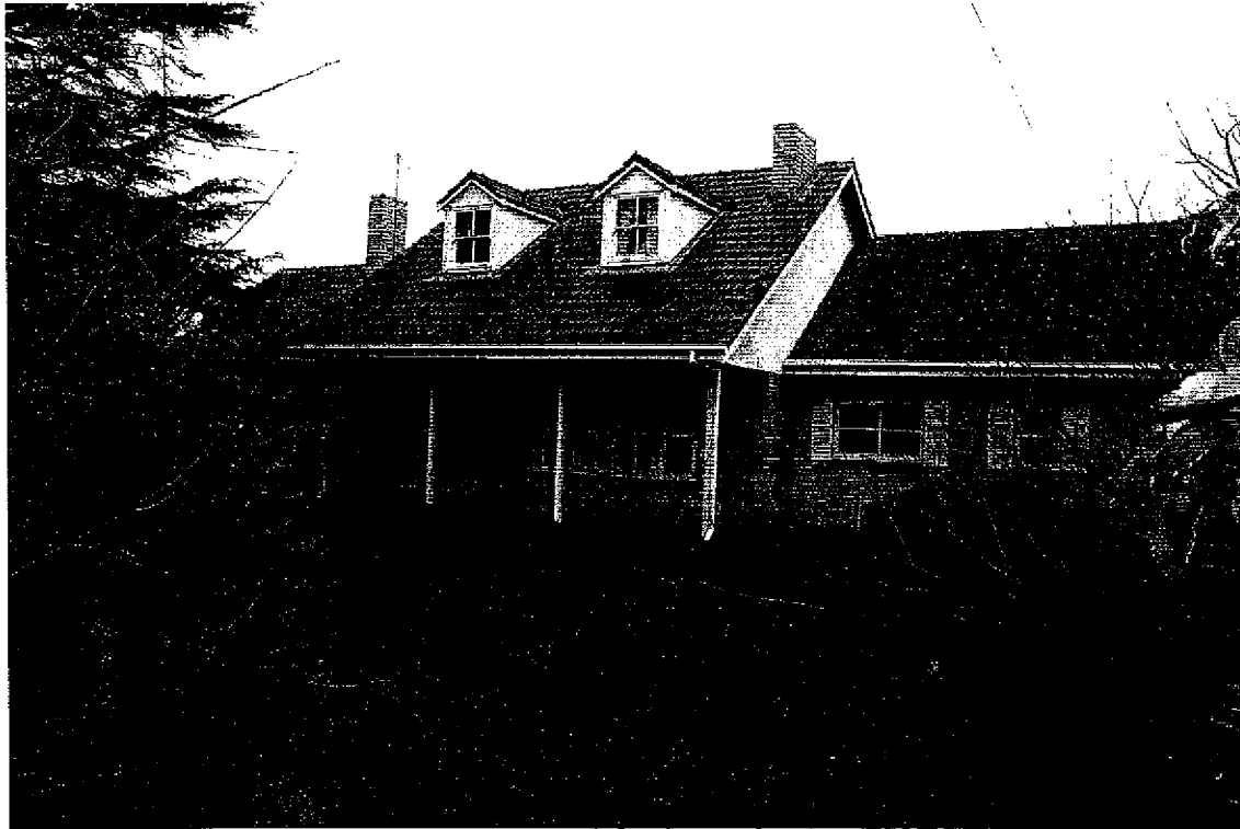
Cuycac Homestead Complex, Chetwynd - Nareen Road, Nareen. Second Homestead
