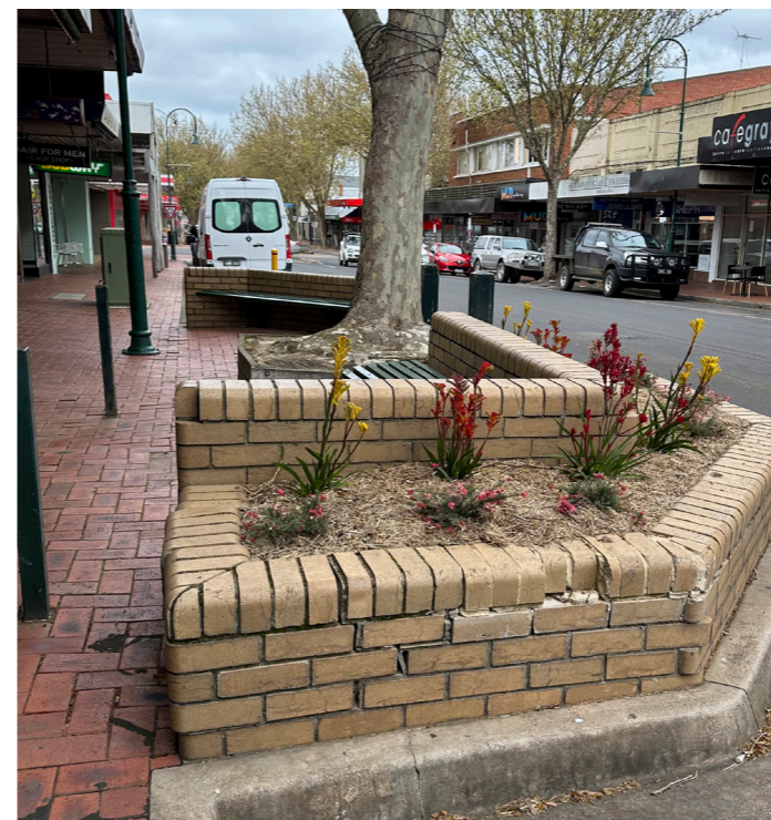
Existing raised planted with brick walling
