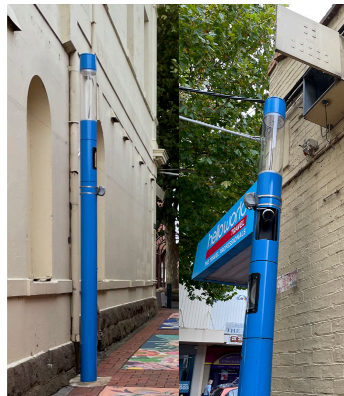
Example of Multi-use pole with lighting and camera - photographed at McGuigan Lane
