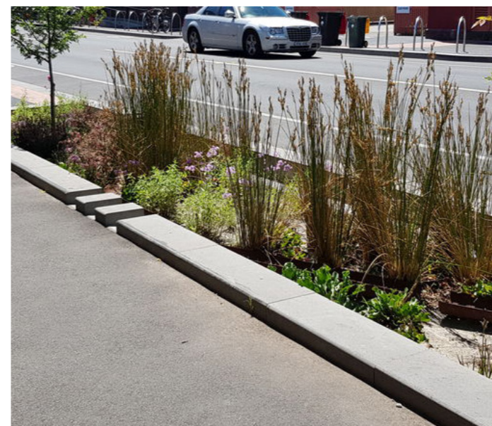
Example of kerb inlet with a layer of stone to dissipate flow.
