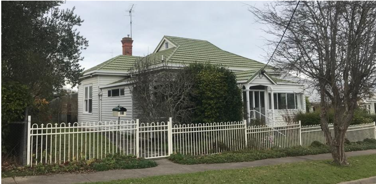
Wrap around verandah built- in on both sides of the gablet
