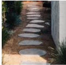
BLUESTONE STEPPERS RECESSED INTO CRUSHED GRANITE SANDS
