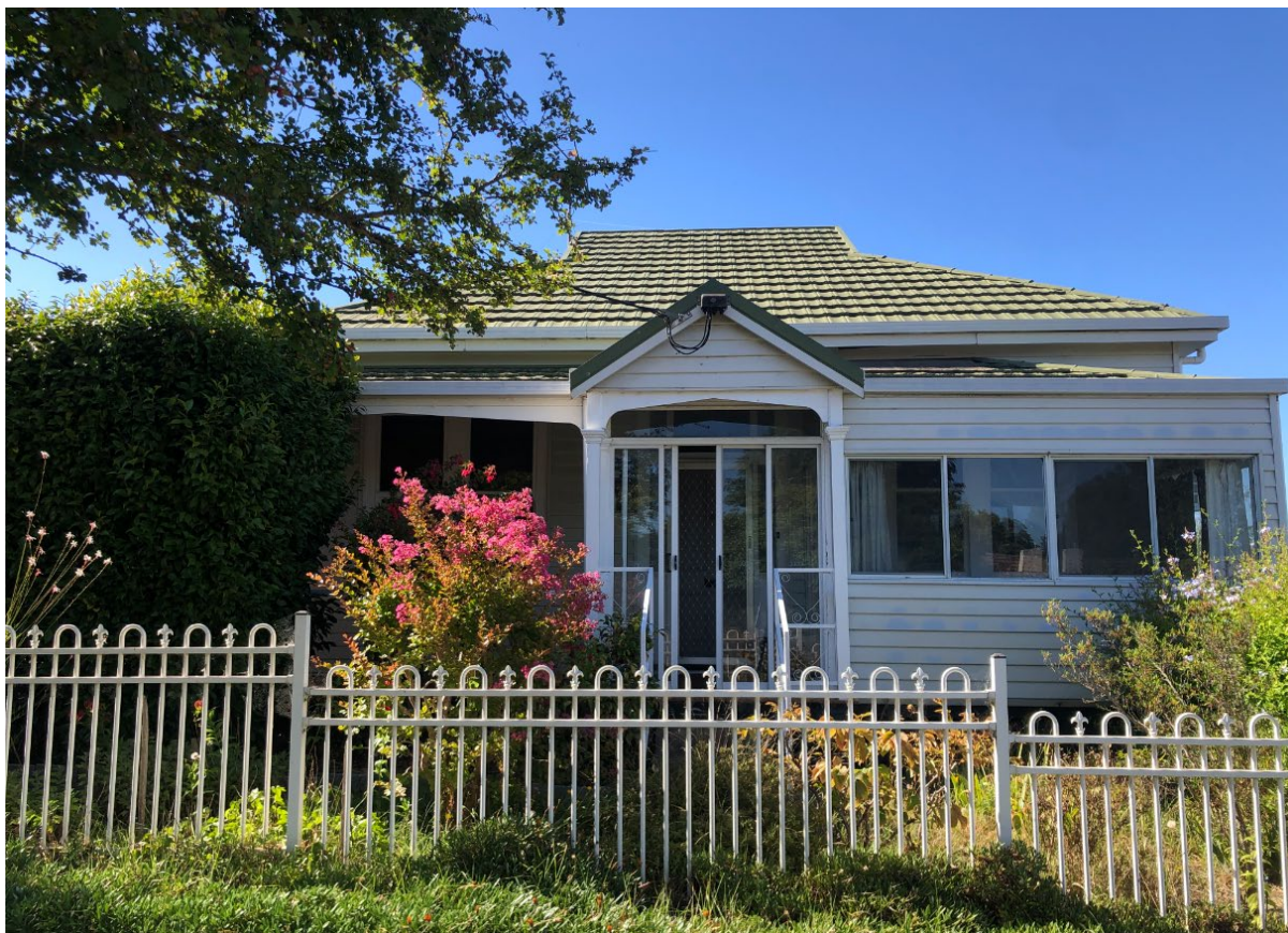
Figure 5 Site photograph taken from Griffin Street 12 February 2024
