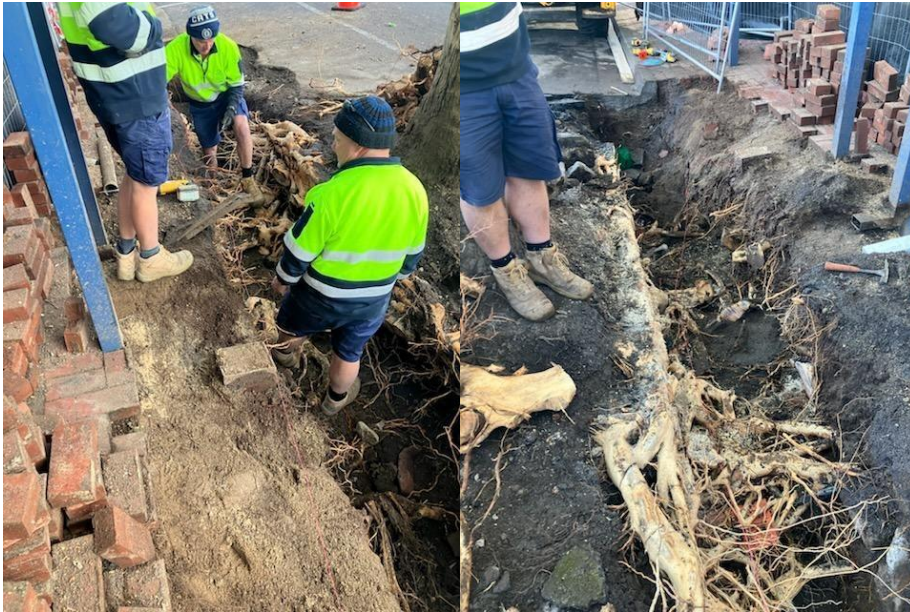
Images of recent kerb reinstatement due to the tree roots of a Plane tree in Thompson Street
