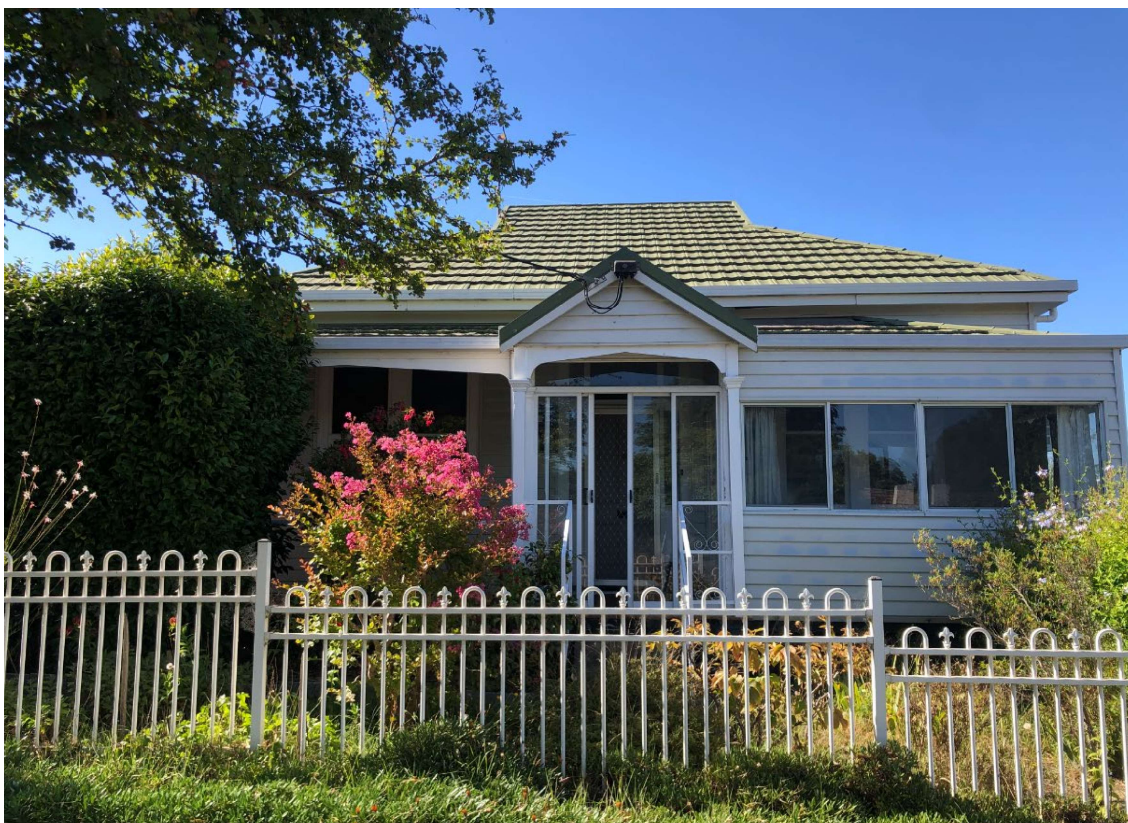
Figure 5 Site photograph taken from Griffin Street 12 February 2024
