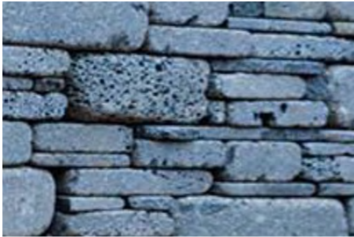
Stone clad wall.
