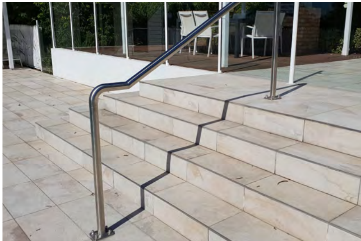
Hand rails stainless steel
